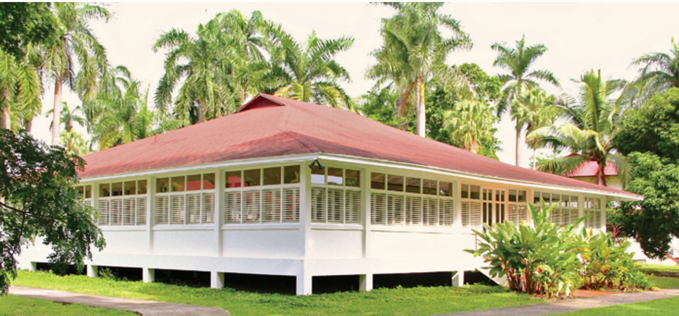
House Museum - Interpretive Center. Above: Architectural elevations for its restoration, made by Architect Eduardo Tejeira Davis.
